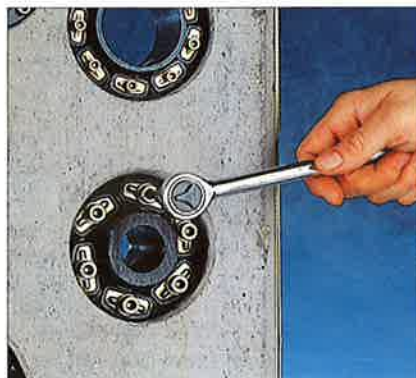
Hexagonal socket head bolts facilitate the assembly of small seal-rings.
